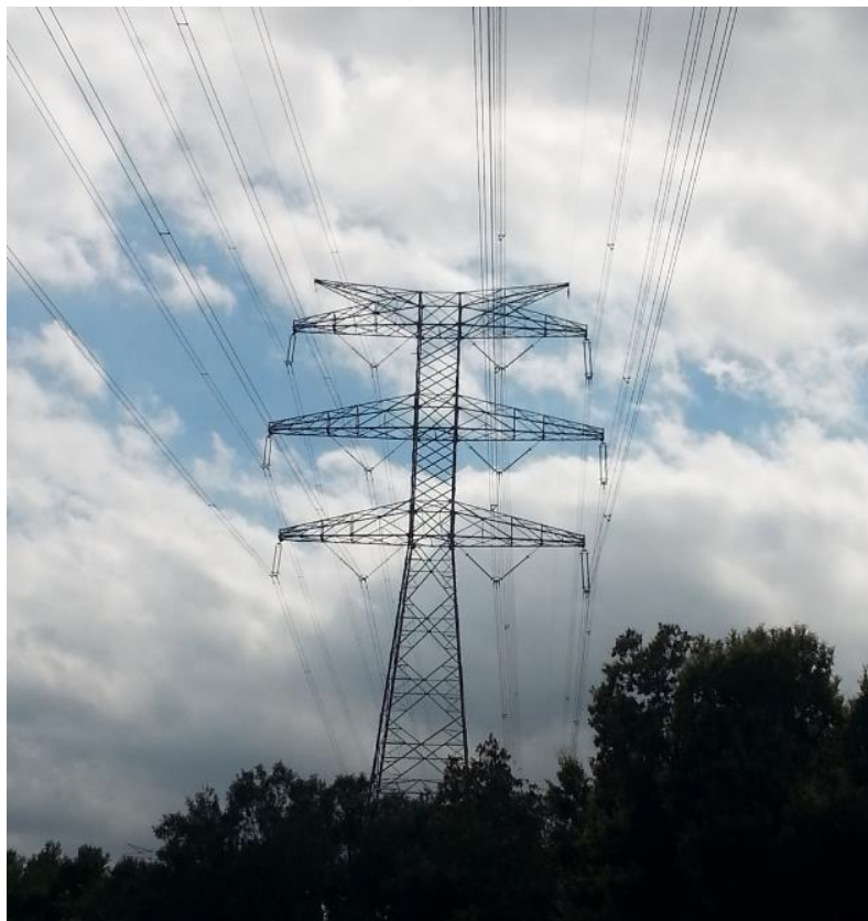
Figure 1. Steel lattice tower
